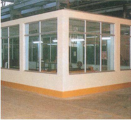
Dust free facility installed for Motor winding.
